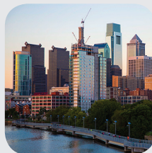
SCHUYLKILL BANKS BOARDWALK COMPLETED
